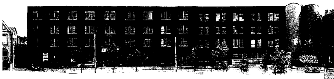
Figure 8 - Viceroy Building, north facade
