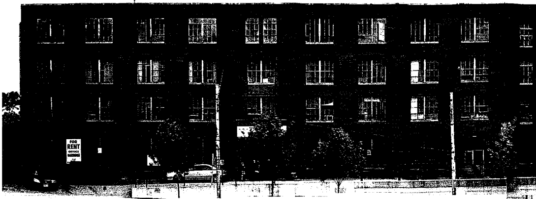
Figure 10 - North Façade – newer east portion – note symmetry and man door at west
