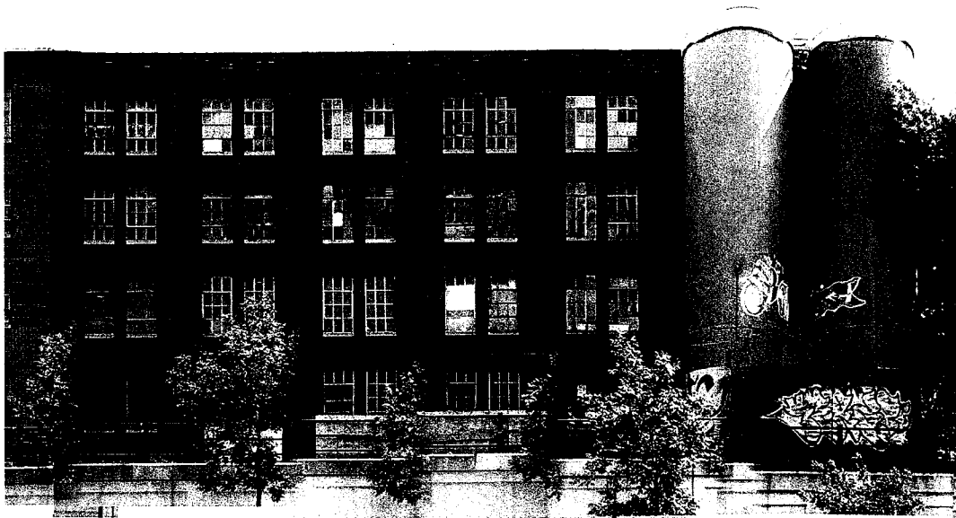
Figure 9 - North Facade – older west portion
