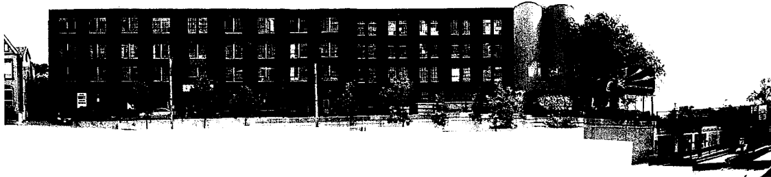
Figure 7 - Viceroy Building, north facade - note transition from commercial to industrial
