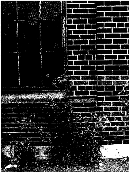
Figure 11 - Dichromatic rug brick, pilaster, steel sash window
