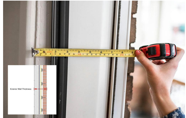
Figure 10 - Measure exterior wall thickness
